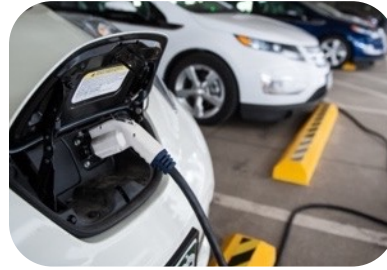
Batteries and Electrification
