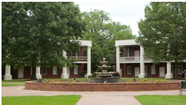
Pentagon Barracks Courtyard
